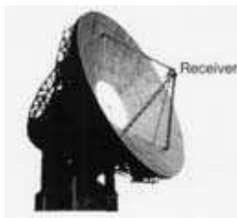
A radio antenna uses metal beams of equal length to support the receiver at its focal point.
